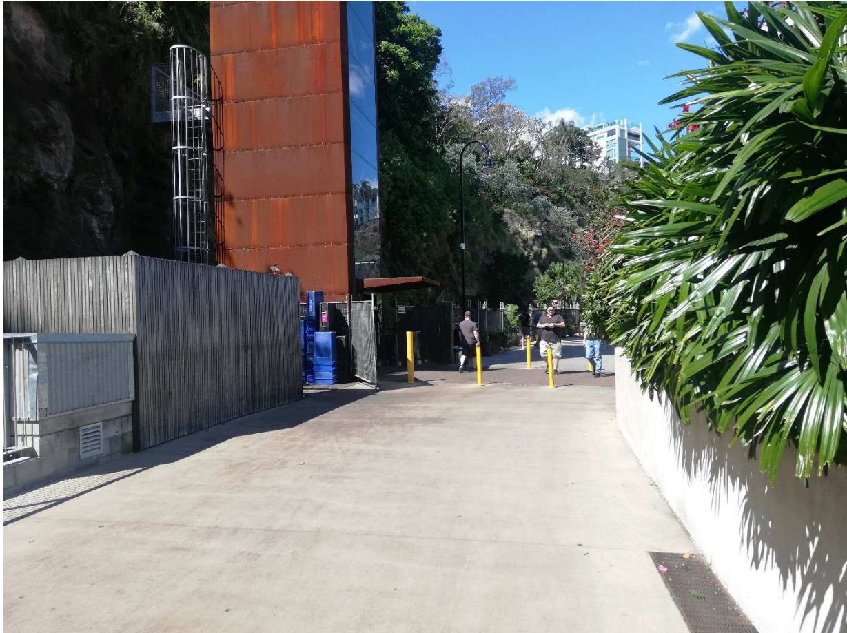
Figure 2: Ground level view of bollard hazard and informal storage with gate typically left open
